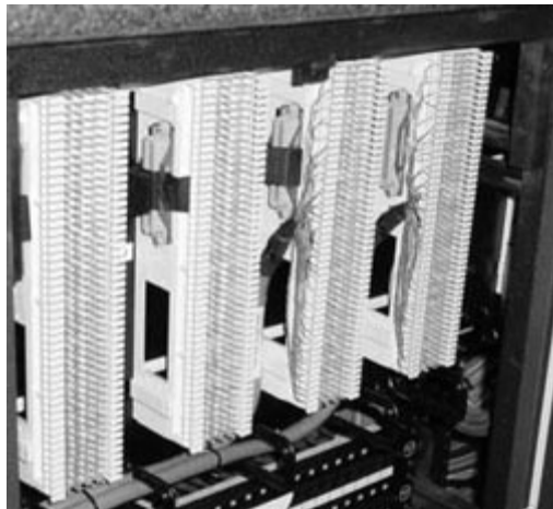
Figure 2 – Wire Connection Blocks
